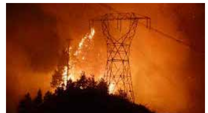
Fire threatening power lines. WA Dept of Transportation
