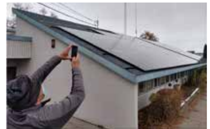
New solar panels on the Nez Perce tribal headquarters in Lapwai, Idaho.
